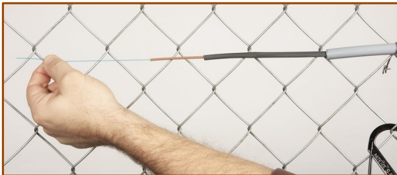
Figure 2-9. End of sensing element with jacket removed and heat shrink, ready for termination.
