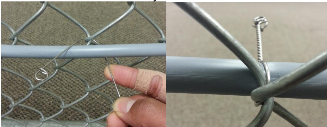
Figure 2-4. Observe how the tie fits tightly within the framework of the fence when correctly routed across horizontally adjacent diamonds
