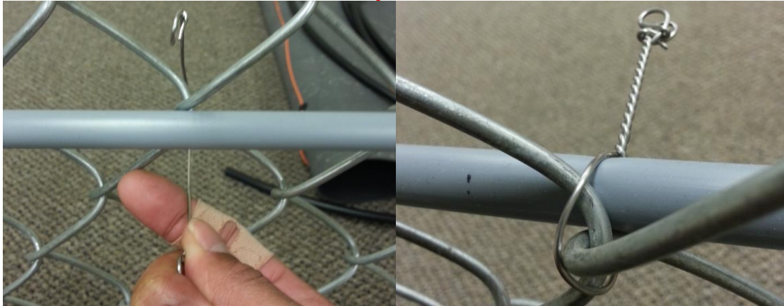
Figure 2-5. Observe that there is not a tight fit when the tie is routed through vertically adjacent diamonds
