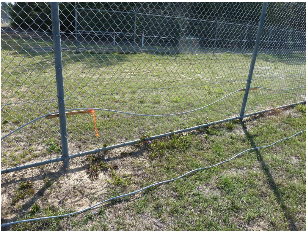
Figure 2-3. Wooden stakes can be used to create a gap between the fence fabric and the fence post to allow for high security routing of the sensing cable.
