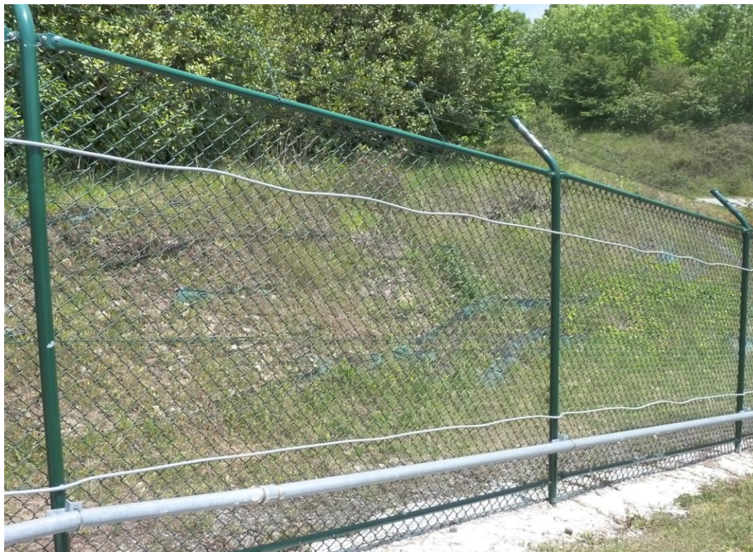
Figure 2-7. Observe the slight bend in the conduit due to hot and cold expansion; more ties and higher tension would prevent this phenomenon
